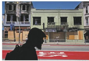
Businesses are seen boarded up in the 3300 block of Mission Street after they were damaged in a fire Saturday that displaced 68 residents and nine businesses, striking at the core of a vibrant neighborhood.
